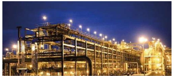
Aramco Jazan Refinery KSA
