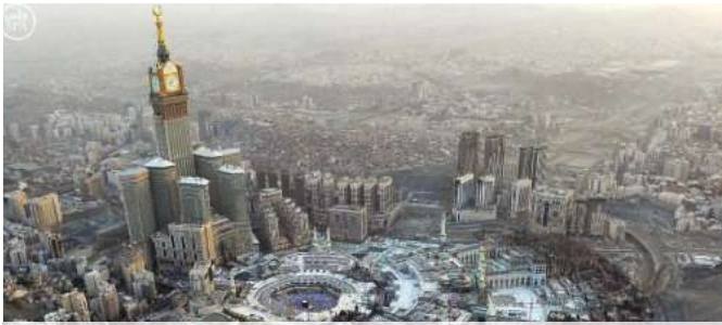
Masjid Al-Haram Expansion Project KSA
